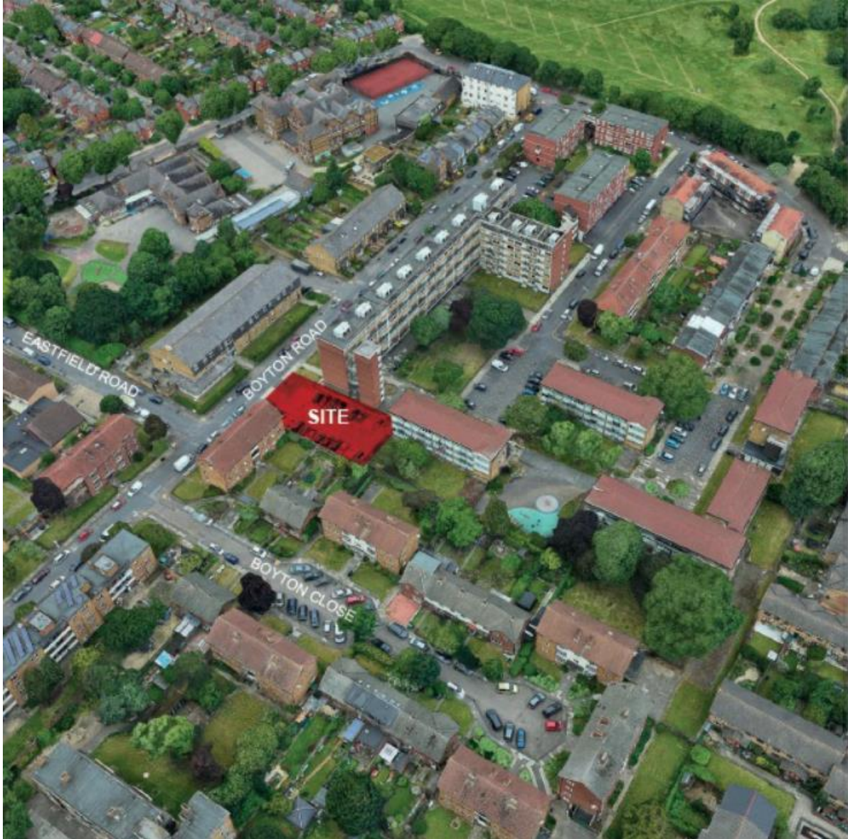
Aerial photograph of site
